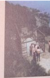
Building the first site hut, 1973
